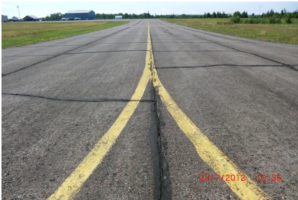
CKC CTA 001 (prior to 2012 rehabilitation)
