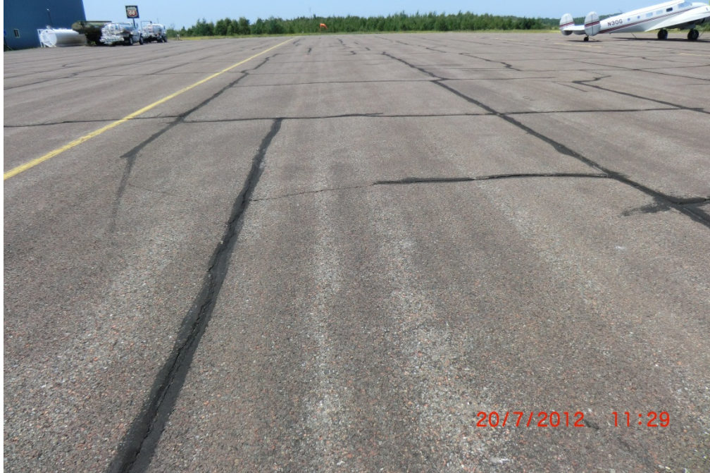
CKC APA 001 (prior to 2012 rehabilitation)
