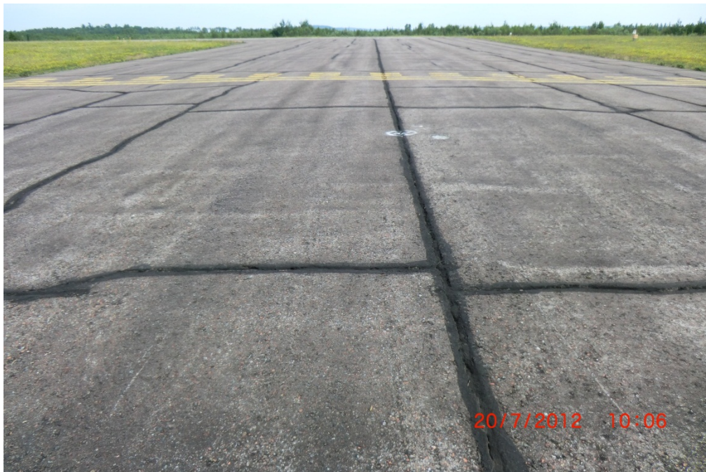
CKC RY927 001 (prior to 2012 rehabilitation)
